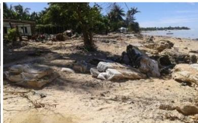
Figure 4: The sea wall that was damaged by the wave
